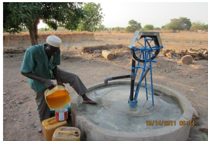
A rope pump installed in the village of Tiogo-Mossi
