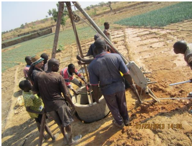
The introduction of a nozzle in a collapsed well in Koukouldi
