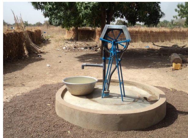
A picture of the same well after USAID WA-WASH intervention. Photo taken on December 18 2012
