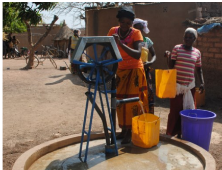
Women take drinking water from an improved well with a rope pump installed by the USAID WA-WASH program.
