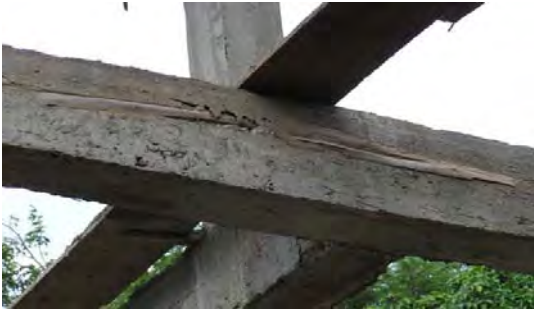
Figure 5: "Honeycombing" - caused by shoddy, cost-cutting construction practices
