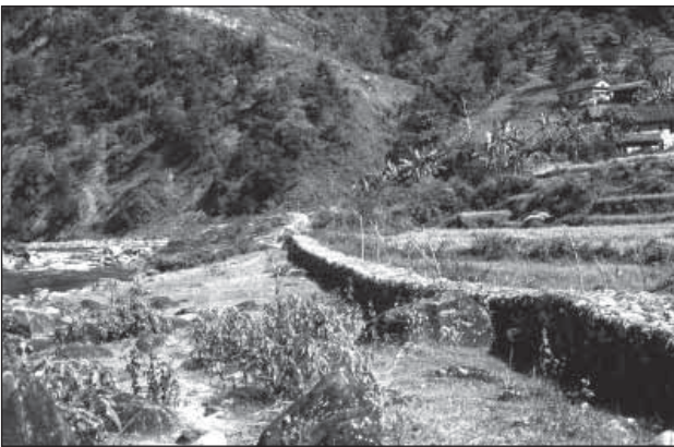
Figure 2. Stone fencing for river control and to keep animals off the farmland.
