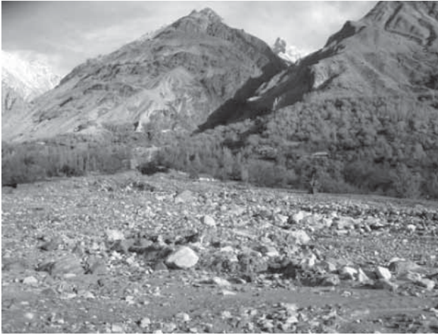
Figure 2. A glacially derived debris flow destroyed 106 houses and large areas of agricultural land in Brep, Chitral District, Pakistan. (Photo: Arun B. Shrestha)
