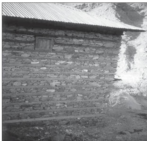
Figure 3. Zinc sheets used as roof
