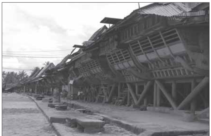
Figure 3. The traditional house in Nias, a time-tested and effective earthquake resistant structure.
