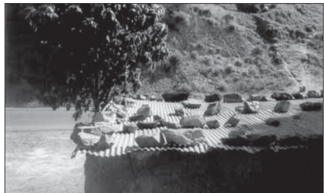
Figure 1. Landslides are common in the area
