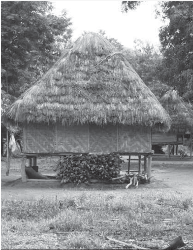
Figure 3. Traditional housing in Singas village – photo depicts housing on stilts, with taller stilts used more regularly today seen on the newer house in the background and the beginnings of a mound surrounded by a drainage ditch in the foreground prior to house building.
