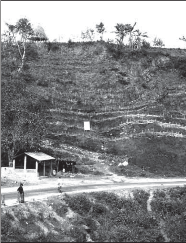
Figure 1. Terrace riser in Tanahu with bamboo matting as landslide protection.
