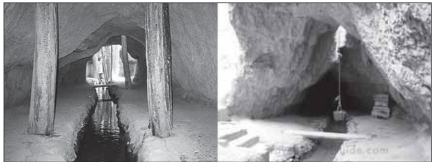
Figure 3. (a) underground canal reinforced with wooden pillars. Source: www.chinahw.net ; and (b) outreach of underground canal to surface canal. Source: www.travelchinaguide.com
