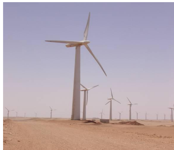
Increased urbanization and pressure on natural resources like water will demand development of alternative energy sources.
