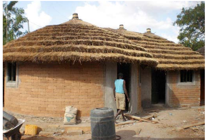
Model tukul (residential hut) made out of cheap environment saving building materials (Photo courtesy of Oxfam GB)
