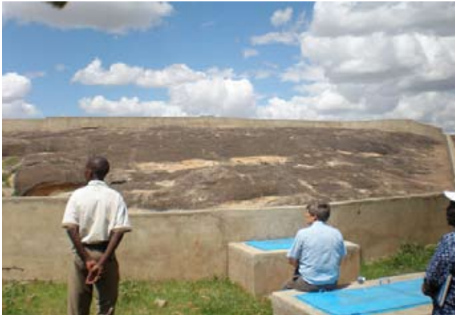
A rock catchment facility in Kotido (Photo courtesy of Oxfam GB)
