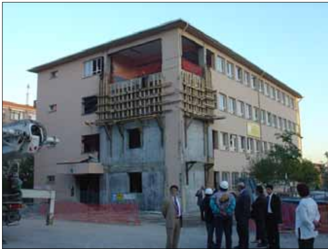
FIGURE 8. Two school buildings under construction in Istanbul. All are completed today. Additional reinforced concrete walls are being added to strengthen the buildings.
