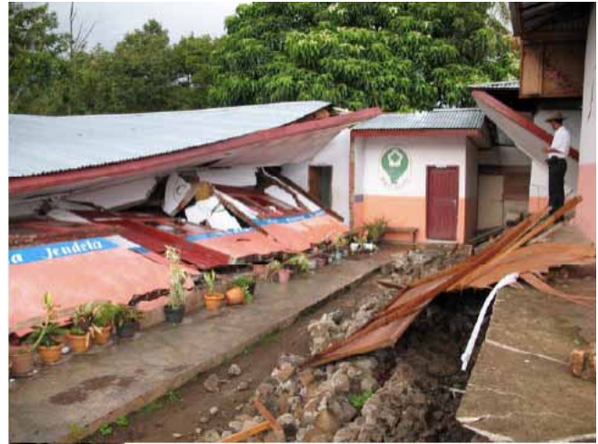
FIGURE 3. A collapsed school near the Sumatra Fault which caused the 2007 M6.3 West Sumatra earthquake. 700 school buildings were damaged in this moderate earthquake, 300 of which collapsed.
