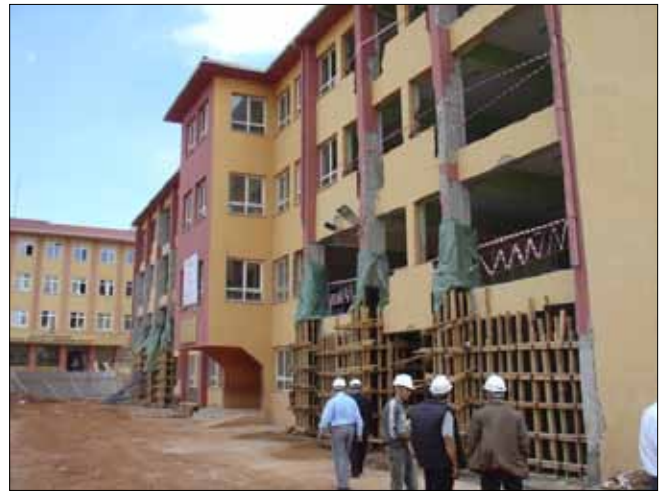
FIGURE 8. Two school buildings under construction in Istanbul. All are completed today. Additional reinforced concrete walls are being added to strengthen the buildings.
