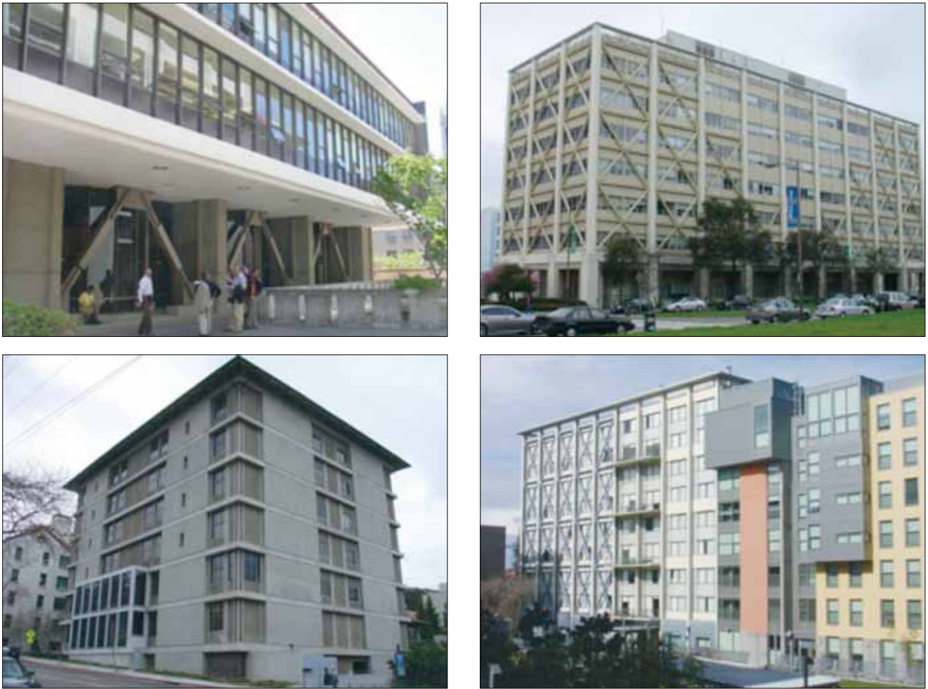
FIGURE 11. Examples of academic, dormitory and administrative buildings that have been strengthened on the Berkeley Campus. Note the various braces that have been added to the facades of the buildings for ease of construction and minimizing the disruption of the interior of the buildings.
