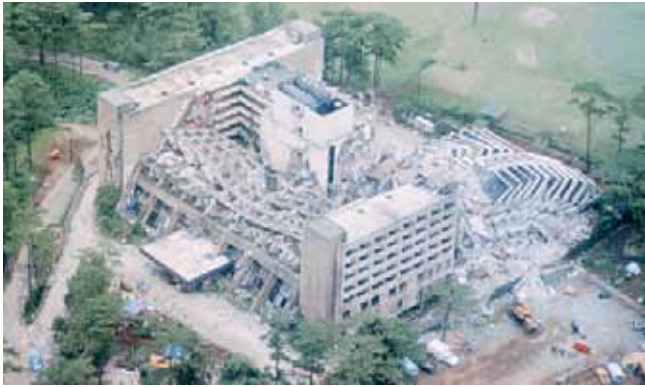
FIGURE 1. One of several collapsed hotels and other modern buildings in the City of Baguio, Philippines; 1990 M7.7 earthquake.
