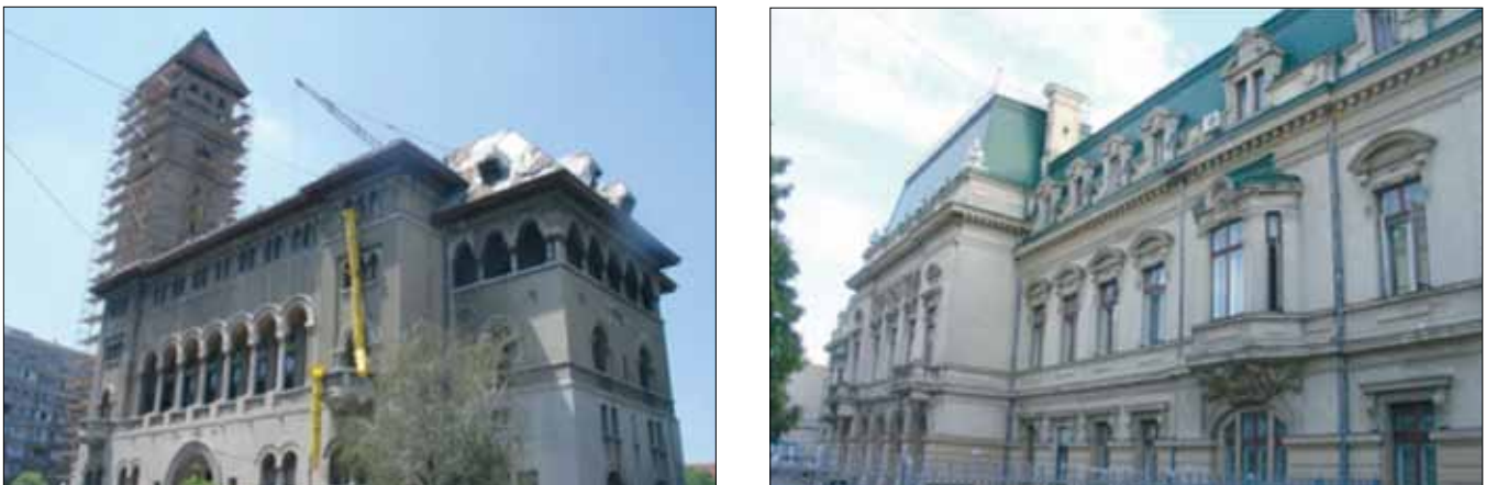
FIGURE 12. Two City Halls in Romania that are currently undergoing strengthening. The one on the left is in Bucharest and has conventional strengthening with reinforced concrete shear walls. The building on the right is in Iasi and will be base-isolated. Both are historical buildings.
