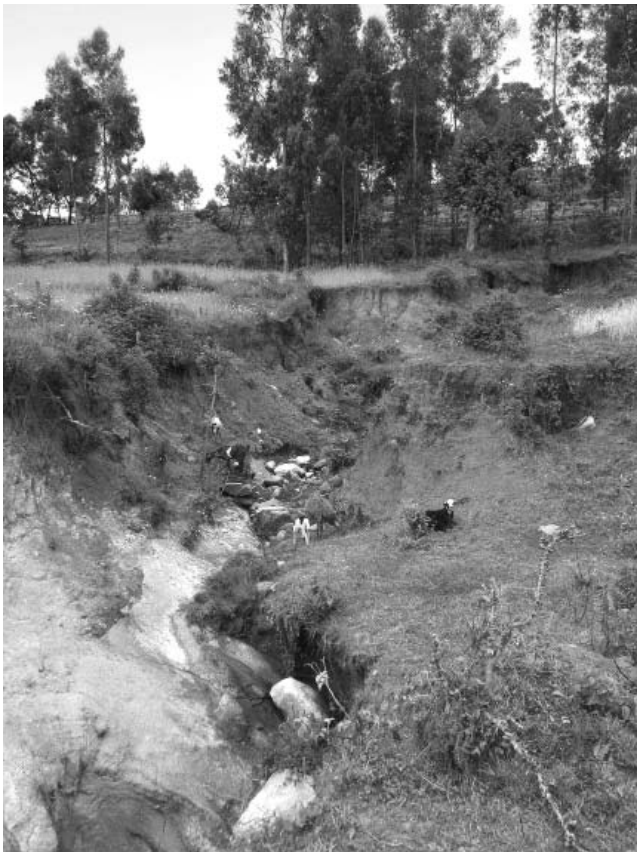
Photo 2.4: A gully caused by soil erosion. Source: Alan Bird
