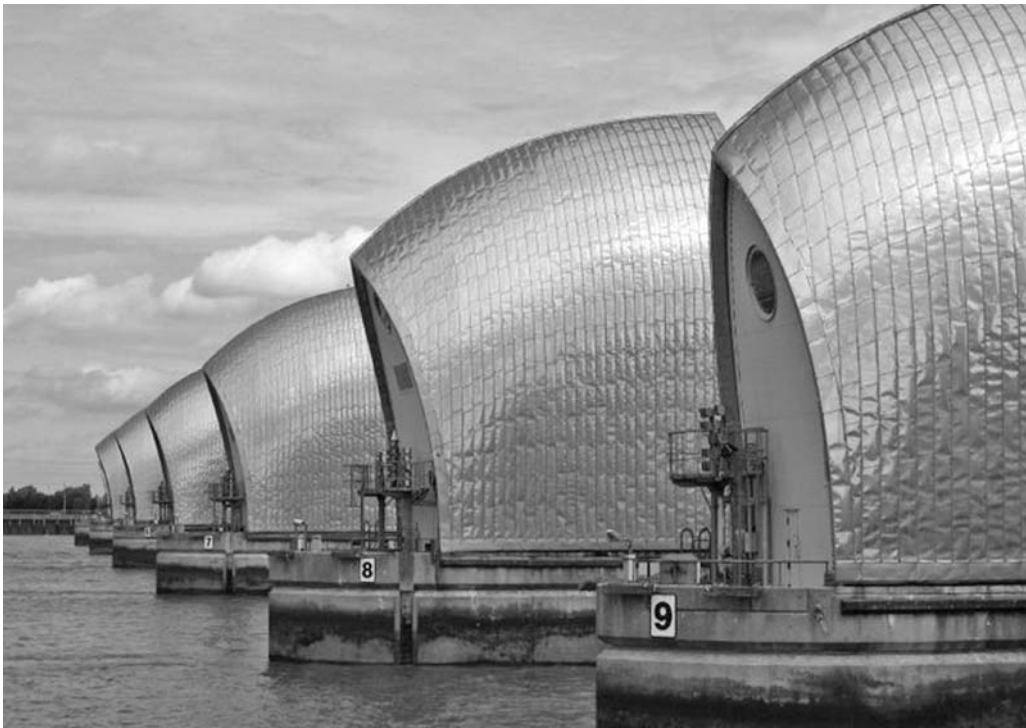
Photo 3.18: The Thames barrier, Source: Nick Dennison
