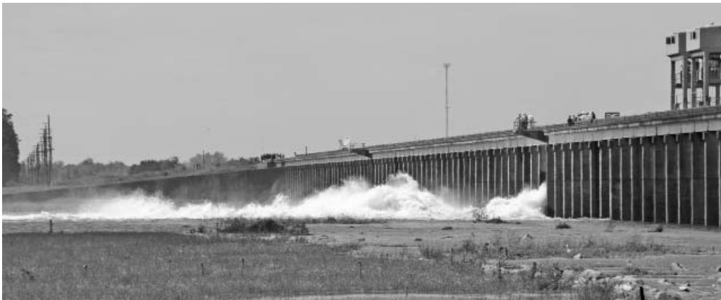
Photo 3.1: The Morganza Spillway opens to divert water from the Mississippi River, May 19, 2011. Source: FEMA, photo by Daniel Llargues
