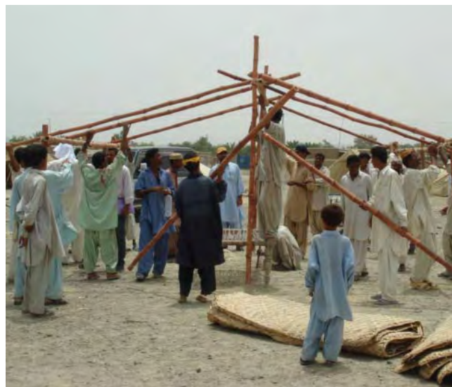
An OFDA-funded program helps cyclone-affected families construct transitional housing in Pakistan (Courtesy of CRS).
