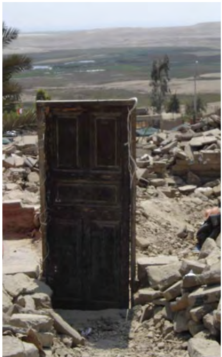
The August 15 earthquake flattened a house in San Clemente District, Peru, leaving only a door in the midst of the rubble (Photo by Alexandra Riboul, USAID).
