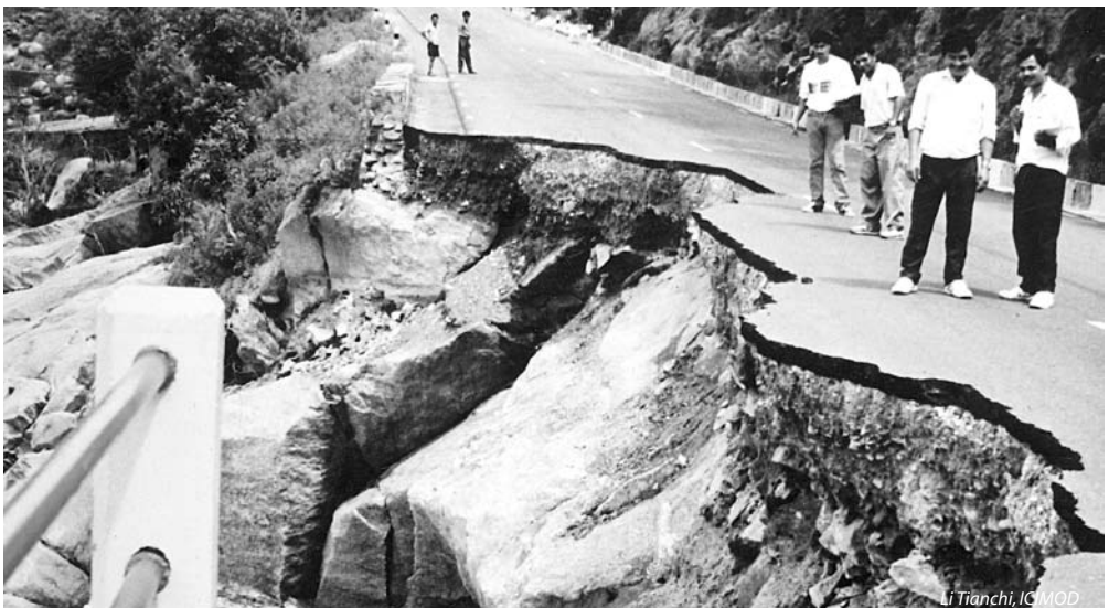
Highway destruction by the floods and landslide each year
