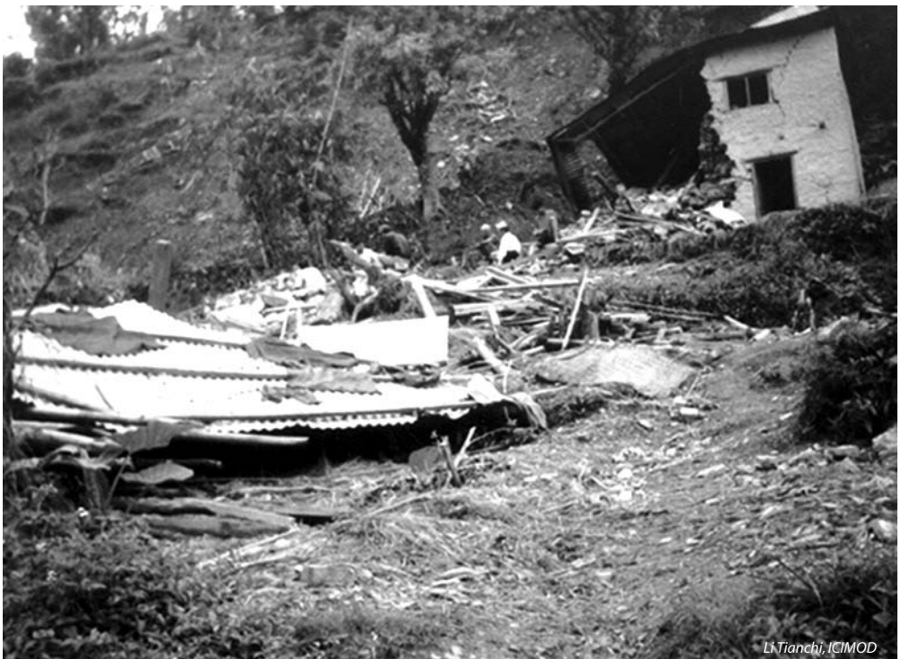
Damaged house by the landslide in mountainous area
