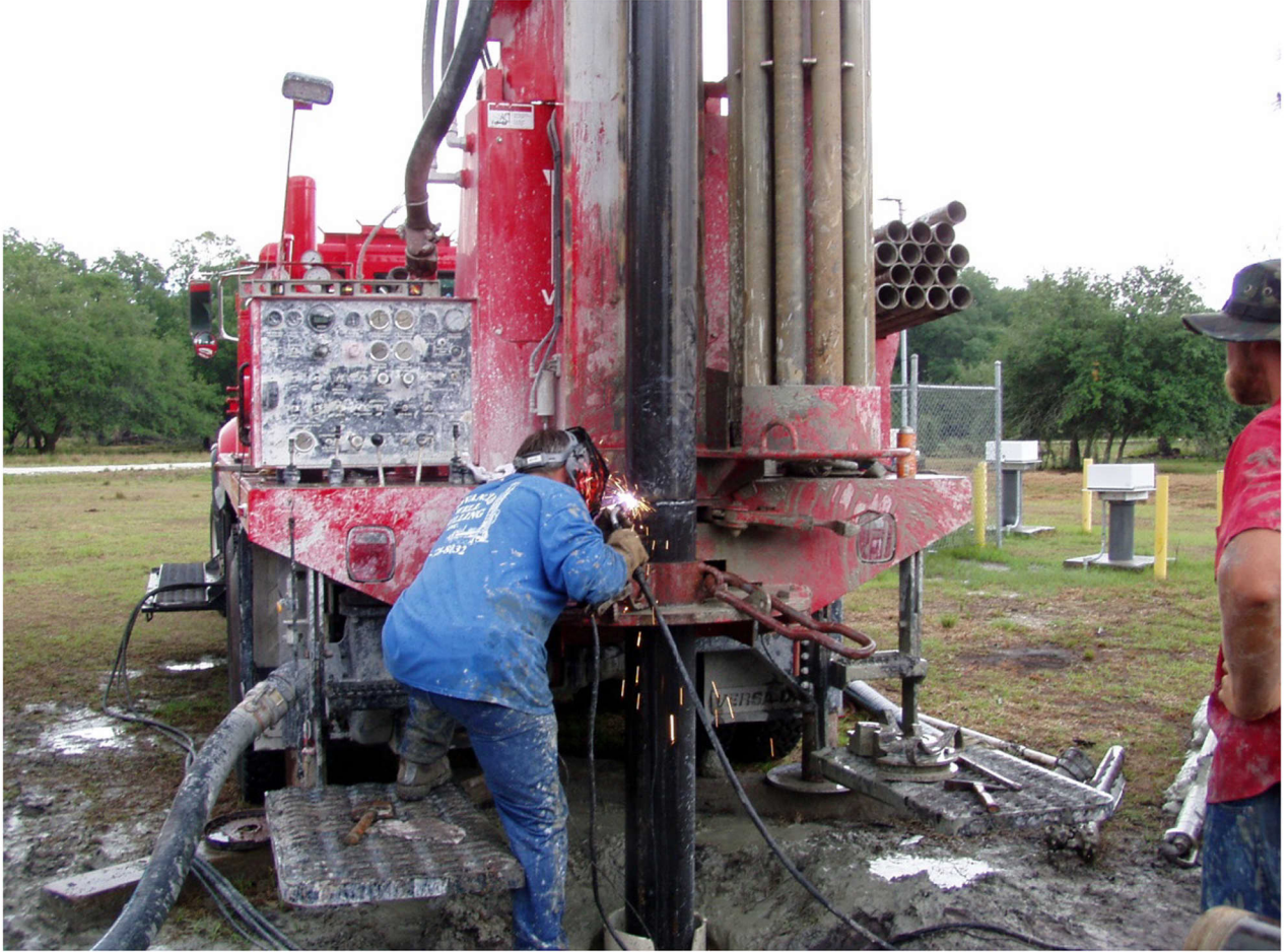
Figure 5. Setting casing at River Ranch site.
