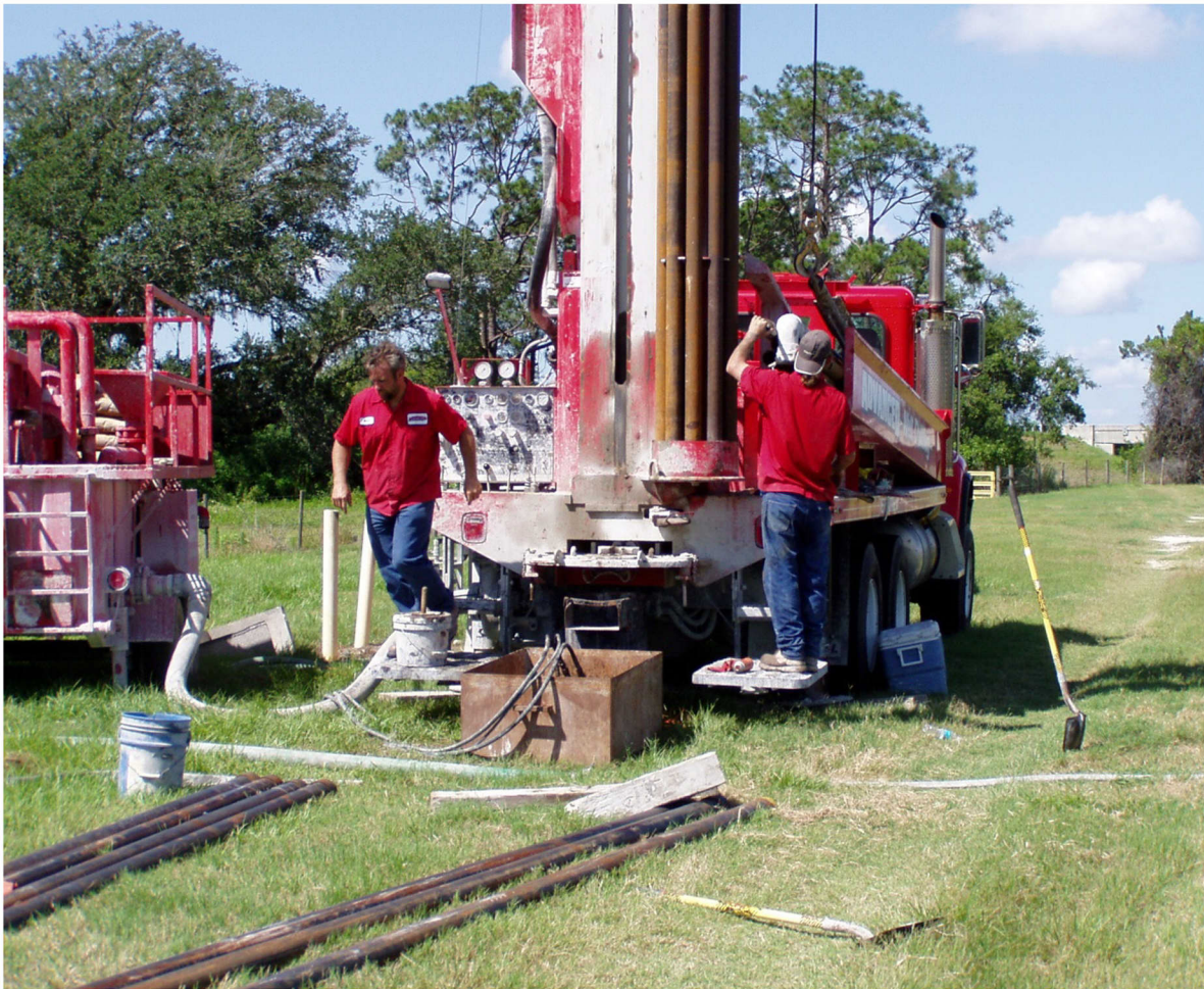
Figure 3. Drilling activities at the St. Cloud site.
