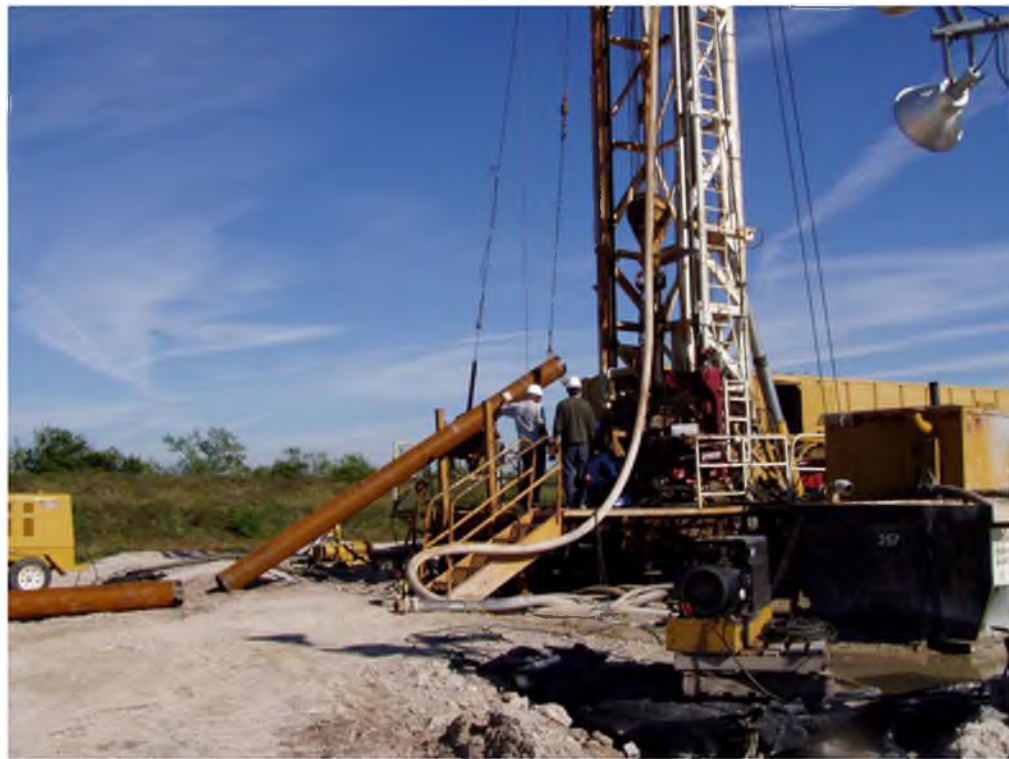
Well Screen Installation
