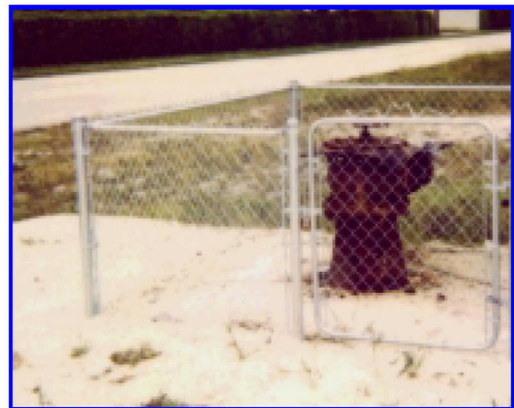
Photo 2: BF-2 (Middle Floridan Aquifer Well).
