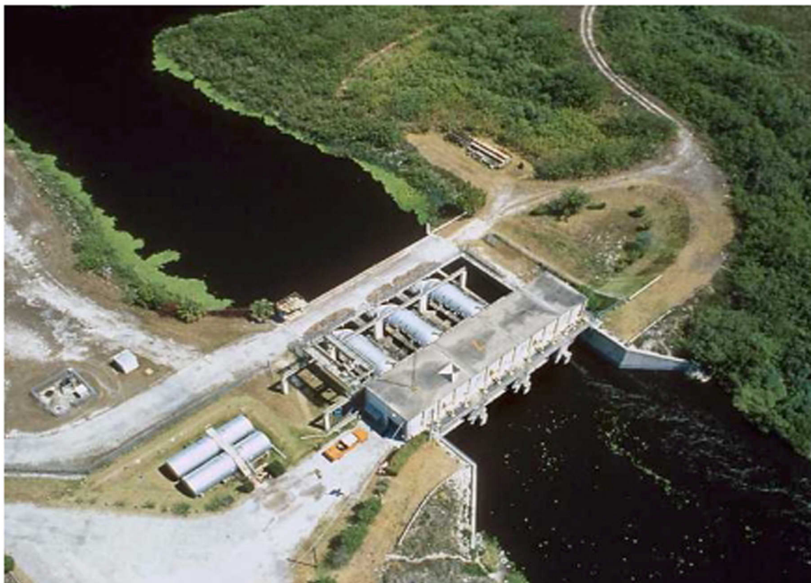
Figure 3. Aerial Photo of S-7 Pump Station from the Southwest
