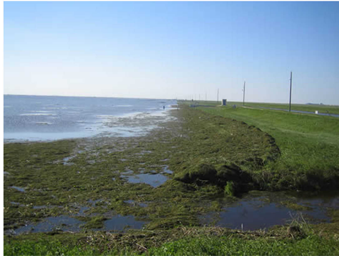
Figure 35. Vegetation pushed by Hurricane Wilma from the interior of the STA to the bank of a levee (photo by SFWMD).
