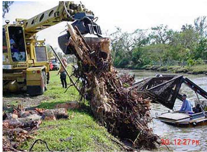
Figure 28. Removal operation of vegetation- and debris-filled canal after Hurricane Wilma (photo by SFWMD).
