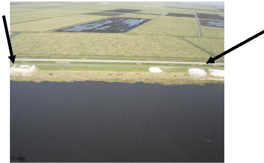
Figure 47. Lake Okeechobee levee damage from Hurricane Wilma (photo by SFWMD).
