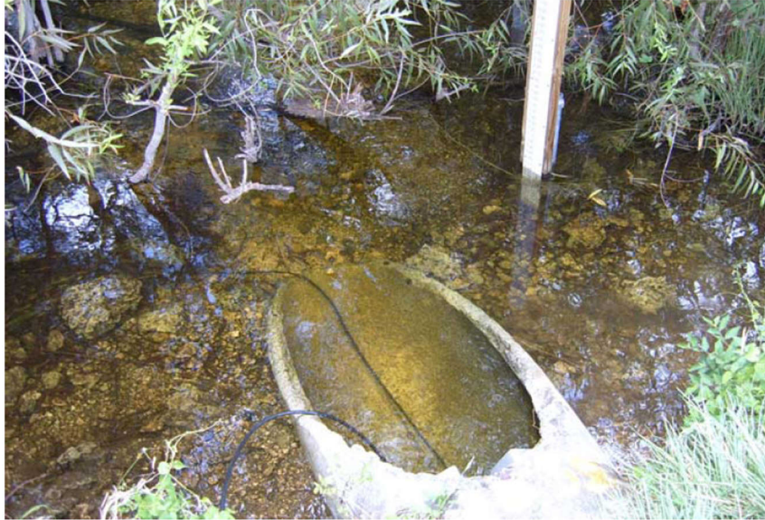
Figure 3 The outlet of Culvert 59— beveled ends
