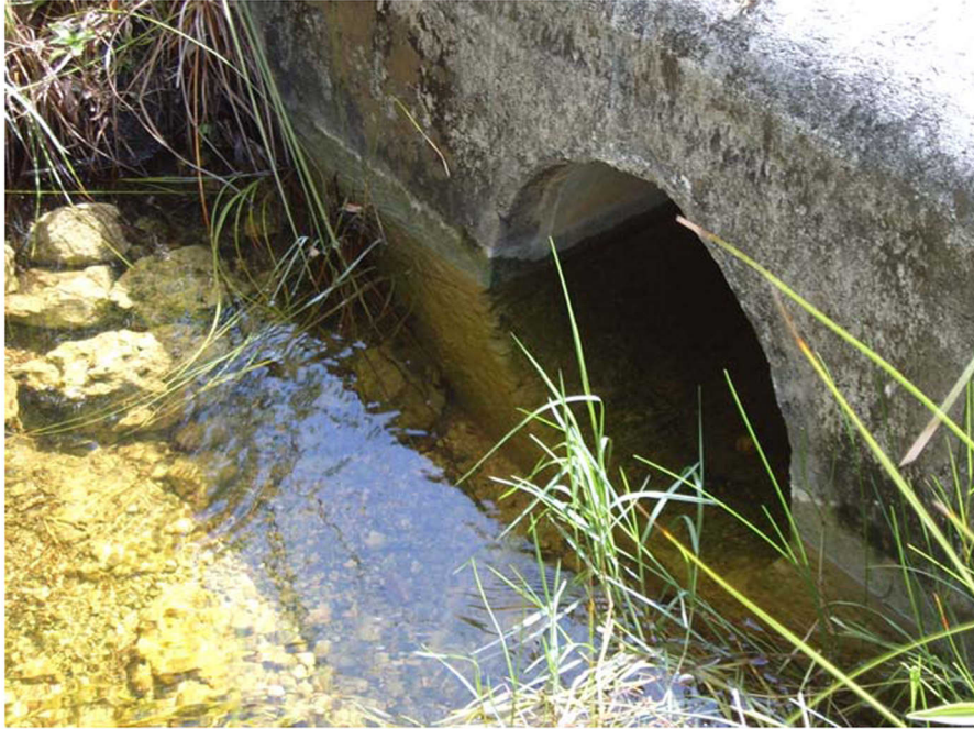
Figure 2 The outlet of Culvert 77 – set flush with vertical headwall
