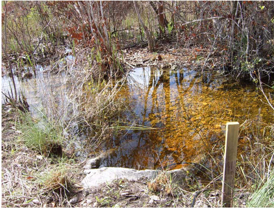
Figure 5 The outlet of Culvert 32
