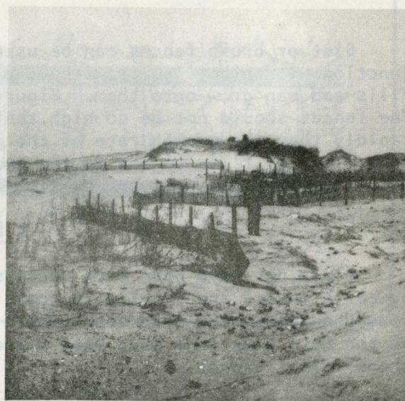
Fig. 47. Sand fences positioned across direction of prevailing wind, also some plantings in this eroded dune field.
