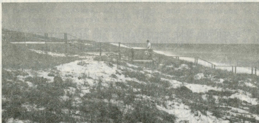
Fig. 34. Good example of board walk between house and beach to prevent erosion caused by people walking over the dunes.
