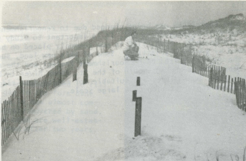
Fig. 39. Two rows of slat fences, the outer straight and the inner undulating, help sand accumulate rapidly.
