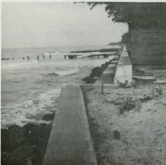
Fig. 13. Beach material loss is due mainly to sea wall and groin structures. No dunes are present to restore with grass plantings, and sand beach renourishment would probably be impermanent.
