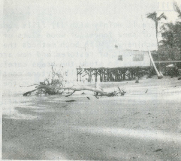
Fig. 37. Beach loss so severe that trees collapse and houses are undercut.
