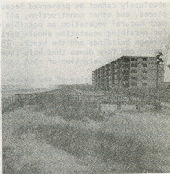
Fig. 36. New construction well positioned behind the second dune ridge with a retaining wall and board walk to the beach.
