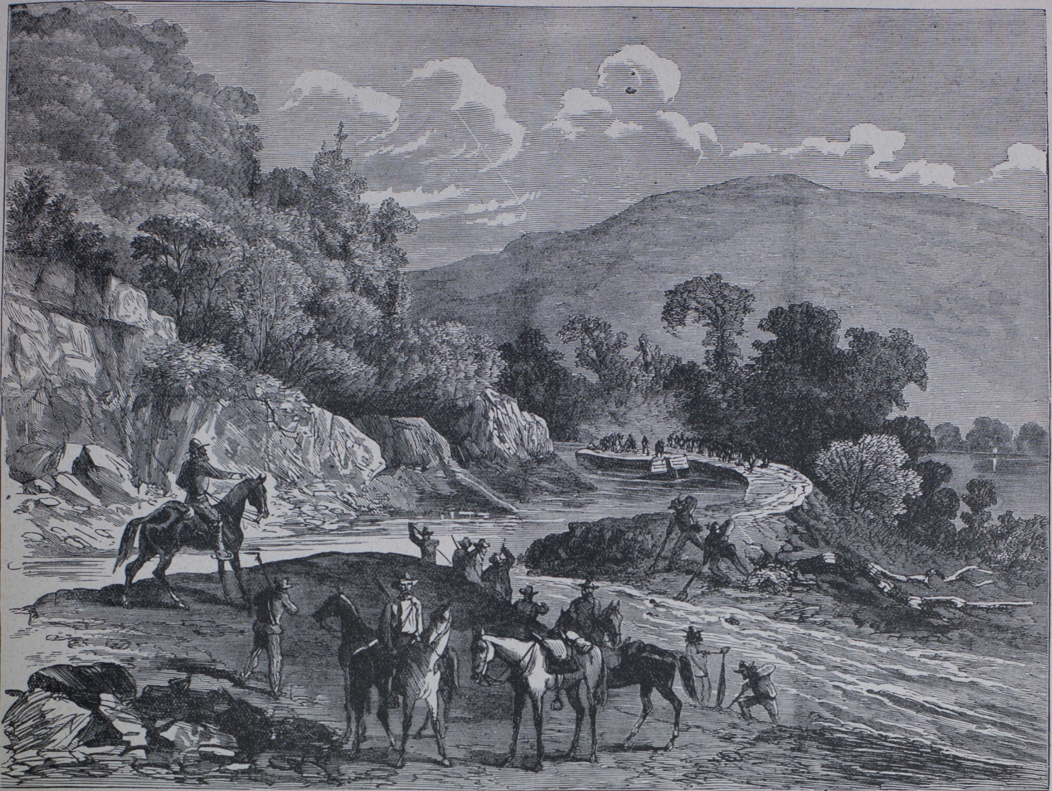
CUTTING THE CHESAPEAKE AND OHIO CANAL.
