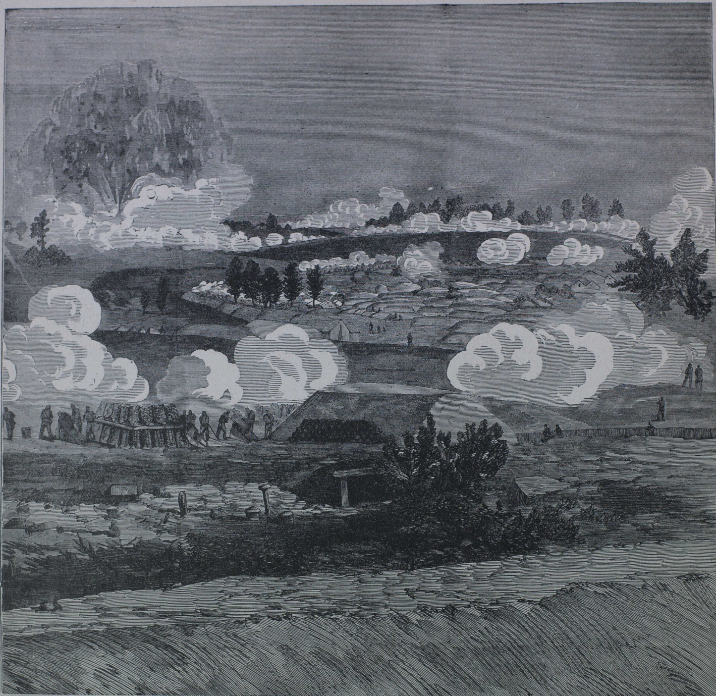
EXPLOSION OF THE MINE.
