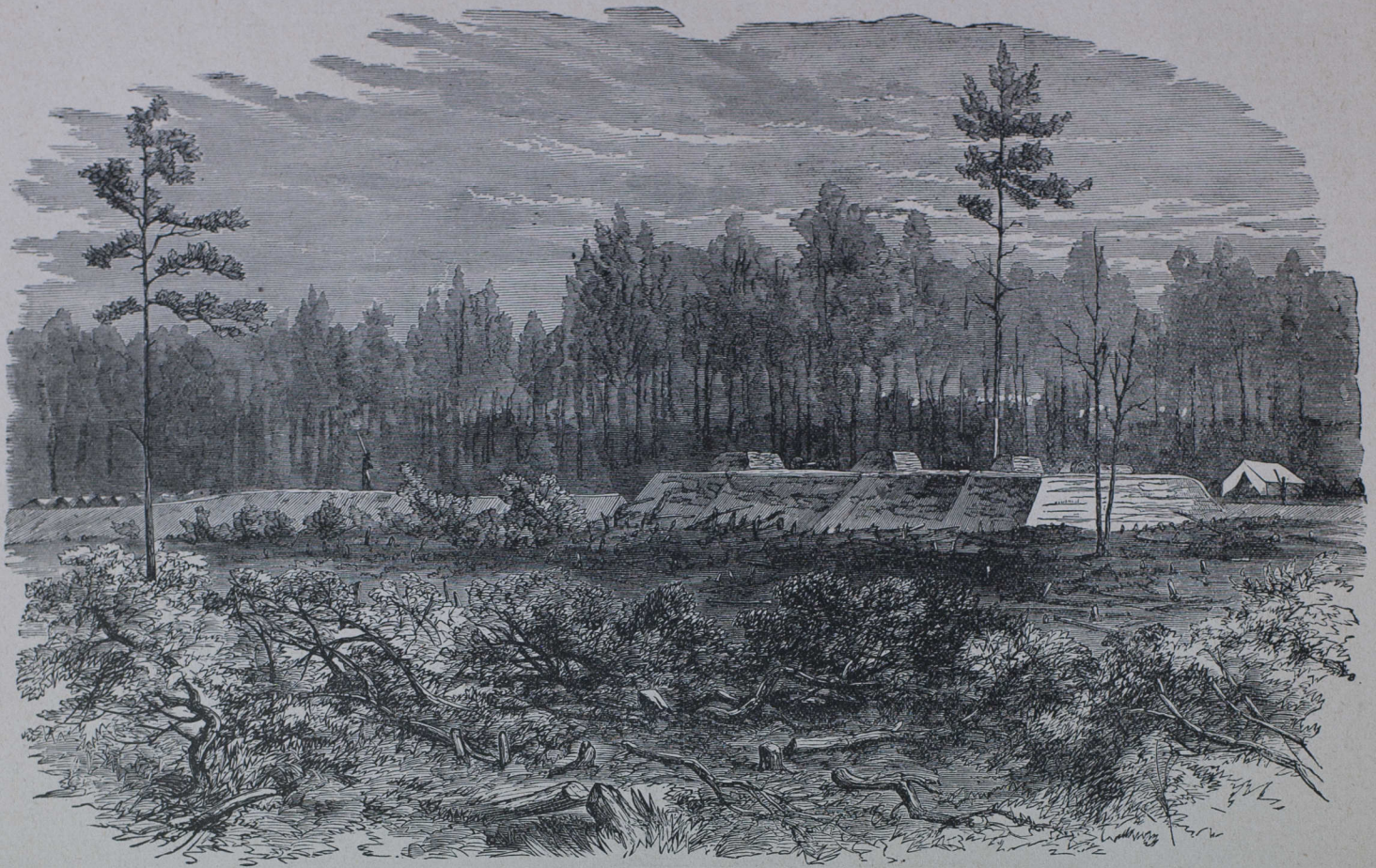
UNION WORKS ON THE WELDON ROAD.
