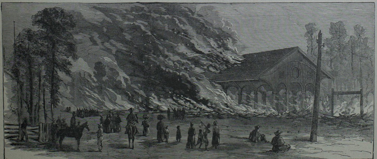
DESTRUCTION OF MILLEN JUNCTION.
