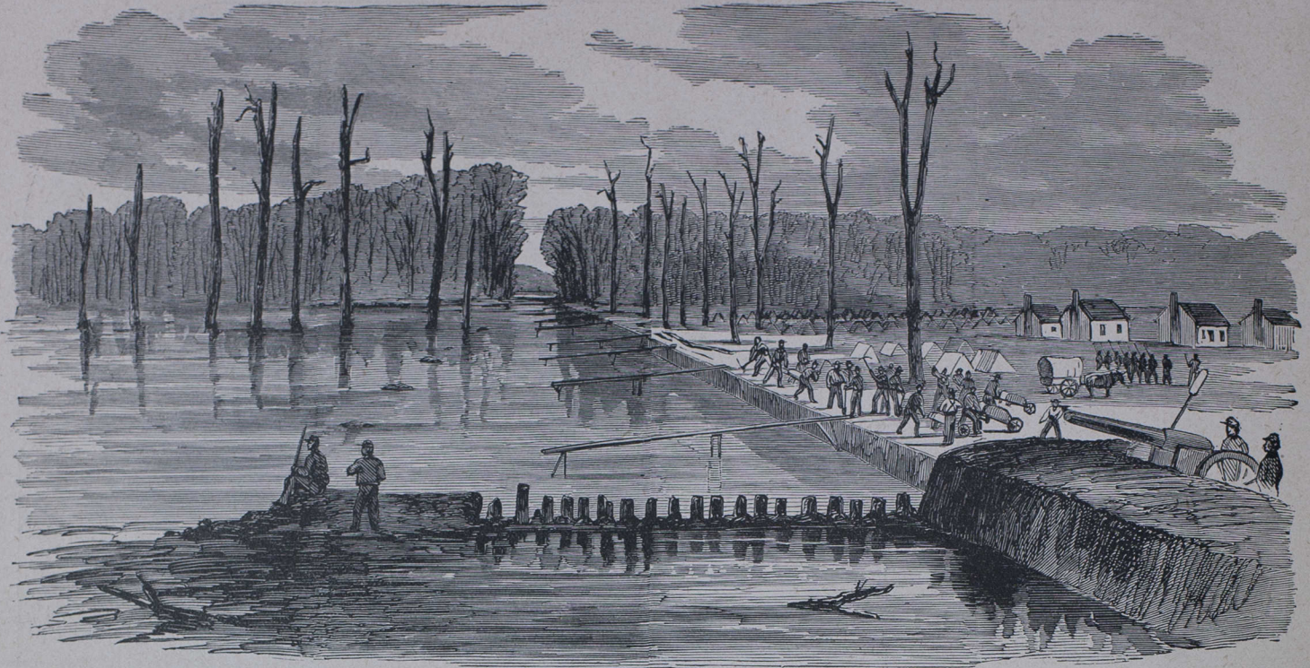
BREAK IN THE MISSISSIPPI LEVEE, NEAR THE CANAL.
