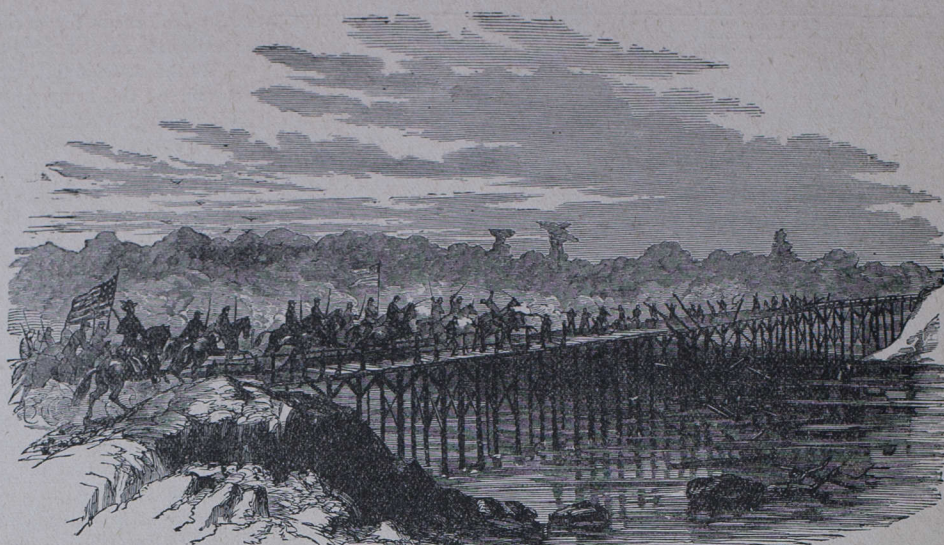
SAVING THE BRIDGE ACROSS PEARL RIVER.
