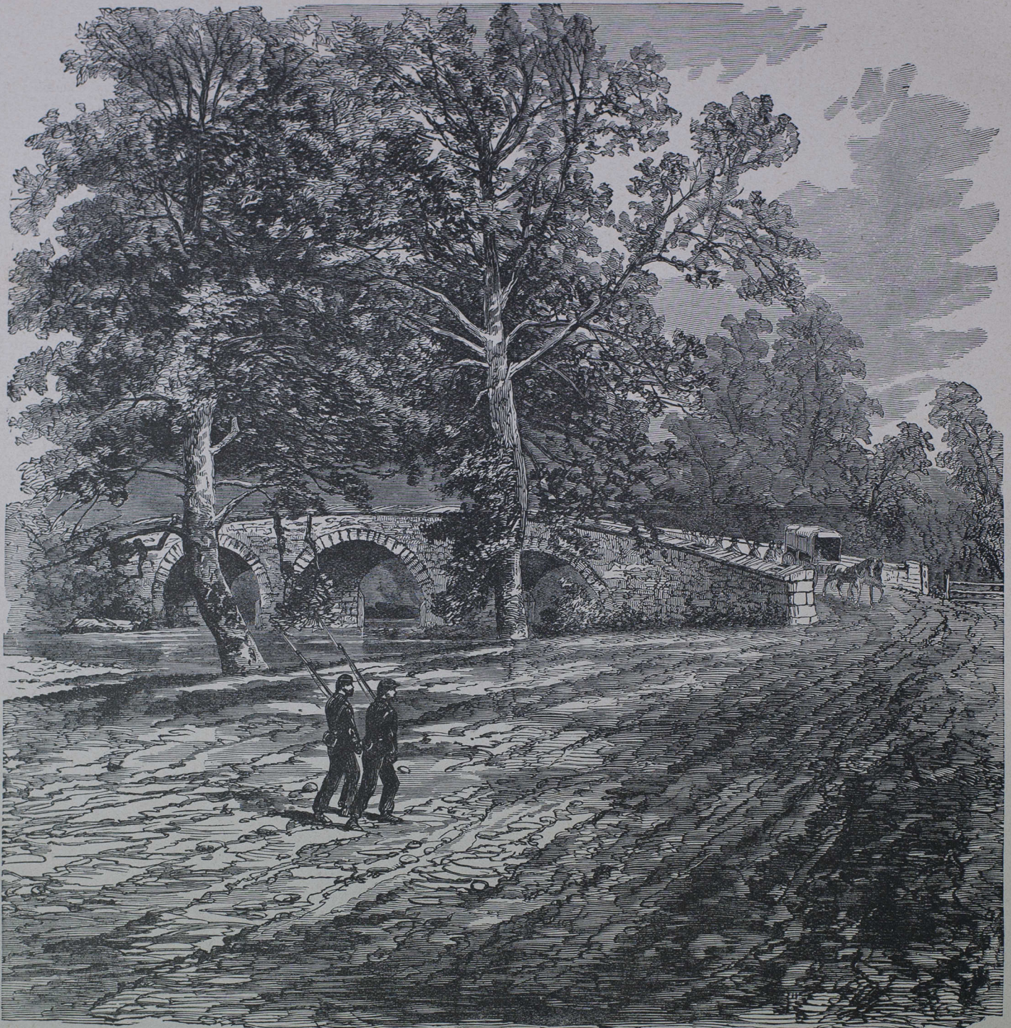
THE STONE BRIDGE OVER THE ANTIETAM.
