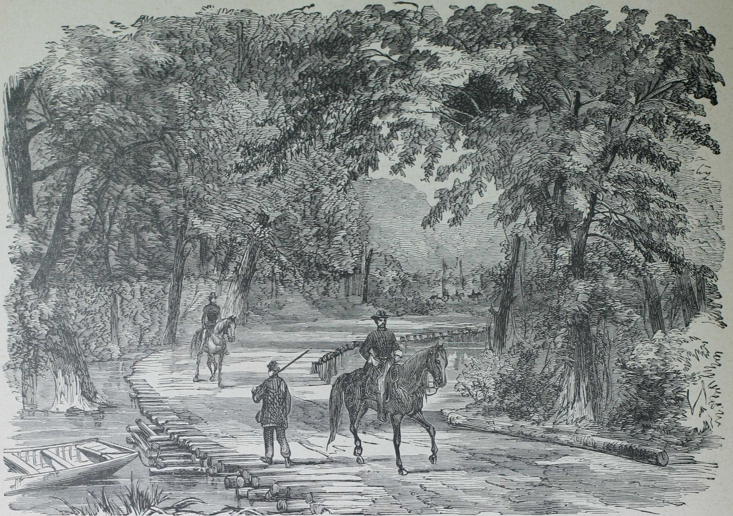
BRIDGE ACROSS THE CHICKAHOMINY SWAMP.
