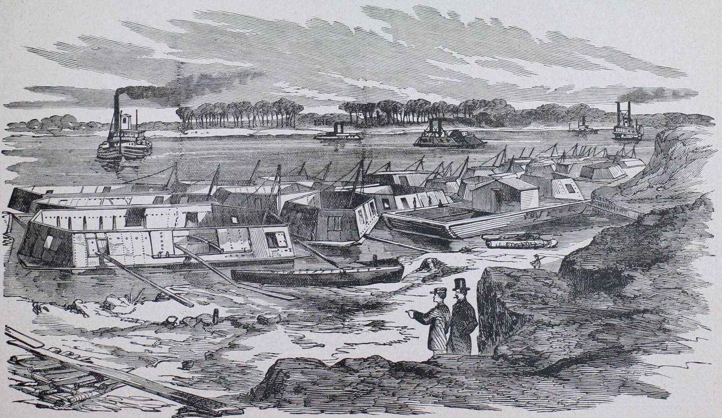
MORTAR BOATS IN PROCESS OF CONSTRUCTION.
