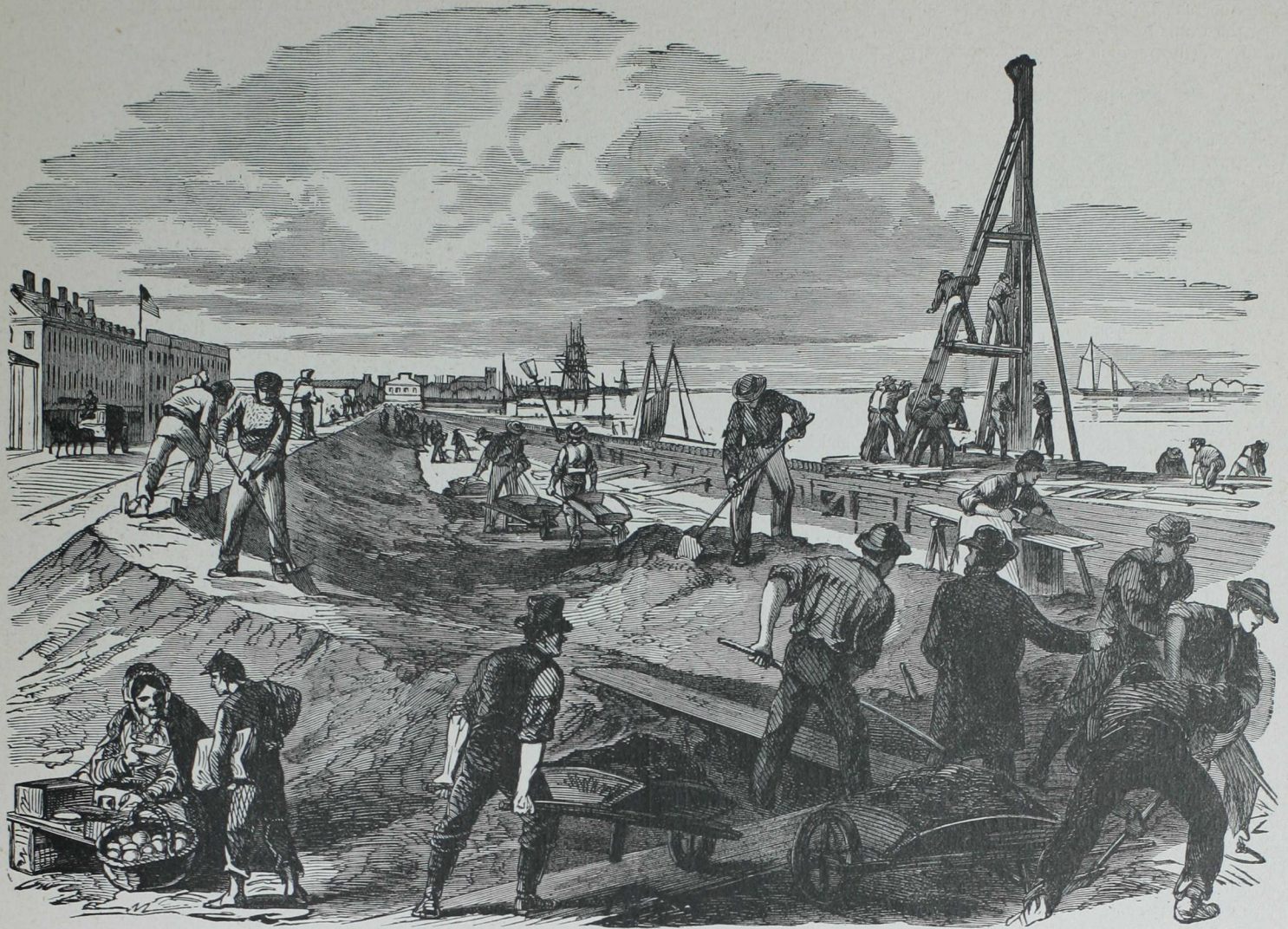
REPAIRING THE LEVEE AT NEW ORLEANS.
