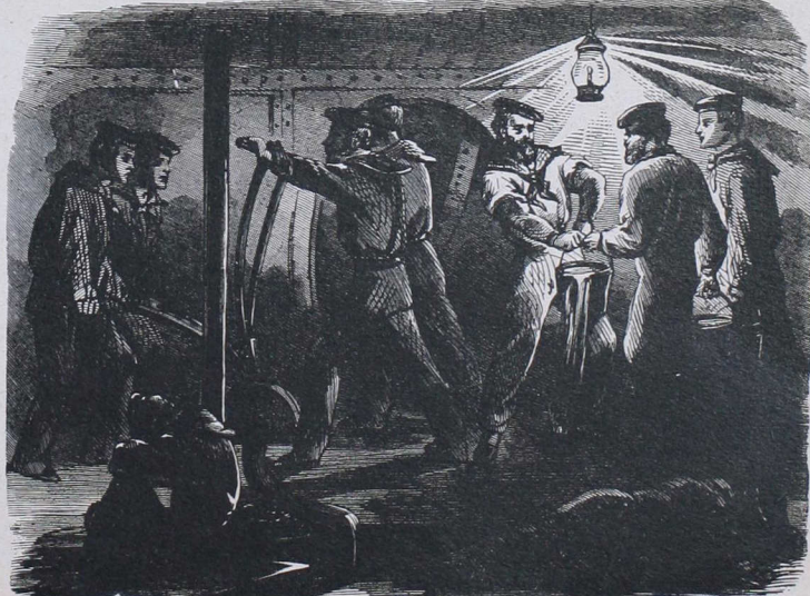
PUMPING AND BAILING.
