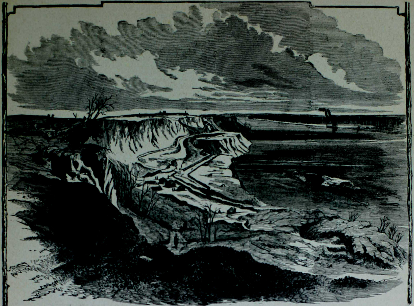
WATER BATTERIES AT COLUMBUS.
