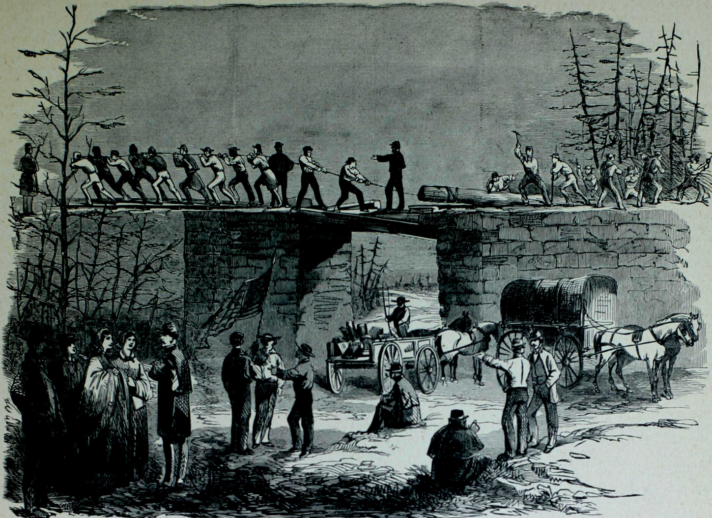
THE MEN OF THE EIGHTH MASSACHUSETTS REGIMENT REPAIRING THE BRIDGES ON THE RAILROAD FROM ANNAPOLIS TO WASHINGTON.
