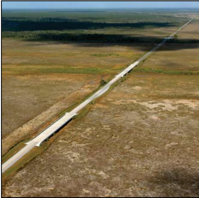
Taylor Slough main flow way and adjacent shorter hydroperiod prairies. New bridges, constructed as part of the C-111 project, have increased the capacity for water conveyance through this area. Photo by William Perry, ENP.
