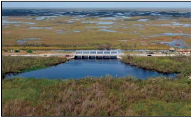
S-12 control structure on the Tamiami Trail. This is one of four structures that deliver water to western Shark Slough, ENP. Photo by William Perry, ENP.
