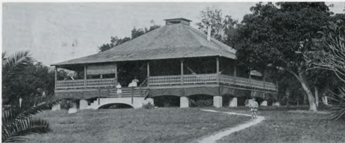
Jessie Munroe is joined by her children in front of the Barnacle. In 1908, the Commodore raised the bungalow and built a cement block first floor underneath. The family lived in Banyan Cottage at Camp Biscayne while the work was progressing. Photo © Munroe Collection, 1977.
