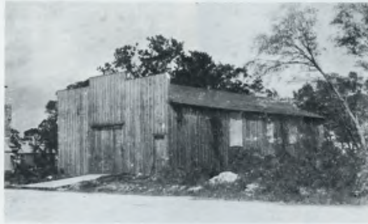
Frank T. Budge operated his hardware store in this unpainted, barn-like structure. The 1901 Dade County Fair was held here at the Budge Opera House. The building later became a bicycle shop. (Photo from the HASF Collection)
