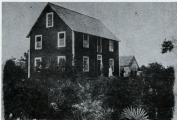
In the early 1900s, William Freeman painted his two story wooden home in Little River with ocher paint he made himself. The clay was gathered from nearby 79th Street. (Photo courtesy of Ethel Freeman West).
