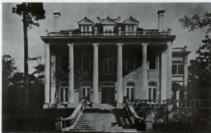
Construction on Hallssee Hall began in 1912. The "Miami stone" used in building the house came from the property, the highest point of land in the city. Walls of the home were 18 inches thick and Hallssee Hall's third floor was a ballroom. Today the landmark is part of the Jackson Hospital Medical Complex. (Photo from the HASF Collection.)
