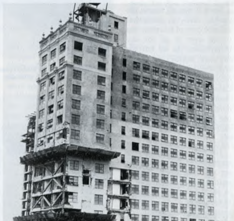
Hit broadside by the wind, the upper stories of the 17-floor Meyer-Kiser building buckled and later had to be torn off. Scaffolding prevented rubble from falling on pedestrians. (All photos: Romer Collection, Miami-Dade Public Library.)
