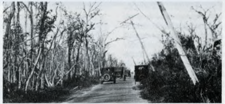
This view of Brickell Avenue looking north from Vizcaya shows damage to the hammock caused by the Hurricane of September 18, 1926.
