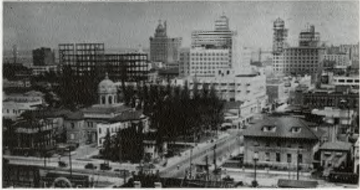
The old Dade County Courthouse saw ironwork pushing skyward during the 1925 building boom.
