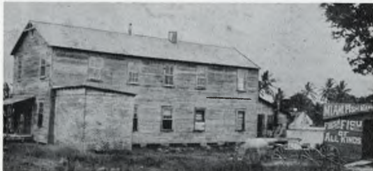
The Dade County courthouse from 1899 to 1904 was a rented frame building on the Miami River, later used as a fish house. The one-story brick structure on the left was added to serve as a vault.
