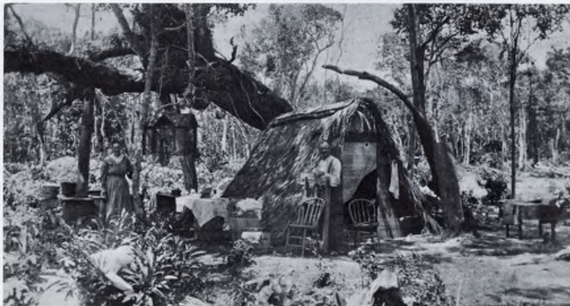
This palm-thatched A-frame with mosquito netting door and outdoor cookstove and pantry was typical of the housing for hundreds of workers who came to Miami during the first boom. In 1896 the population went from near zero to 2,000. — HASF Museum collection.
