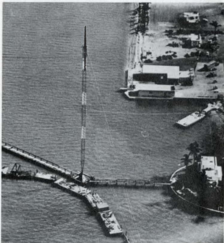
One of the present WIOD towers being erected on North Bay Causeway, 1950. Note the open bay around tower before being filled in for Channel 7 and present WIOD building. —Photo courtesy Radio WIOD
