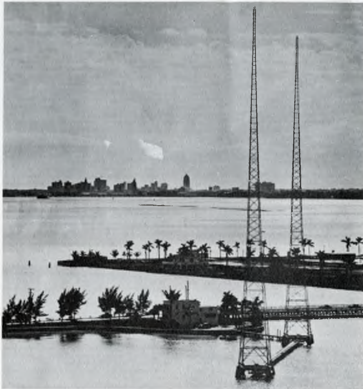
The WIOD directional antenna system and 5000-watt transmitter site, North Bay Causeway, 1941. Portions of the Bay were filled in 1956 to form the site now occupied by studios, offices, and transmitter site. Both towers have since been replaced because of hurricane destruction. —Photo courtesy Radio WIOD
