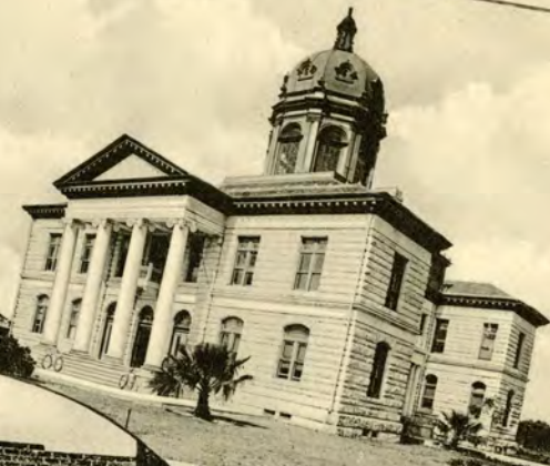
DADE COUNTY COURT HOUSE
