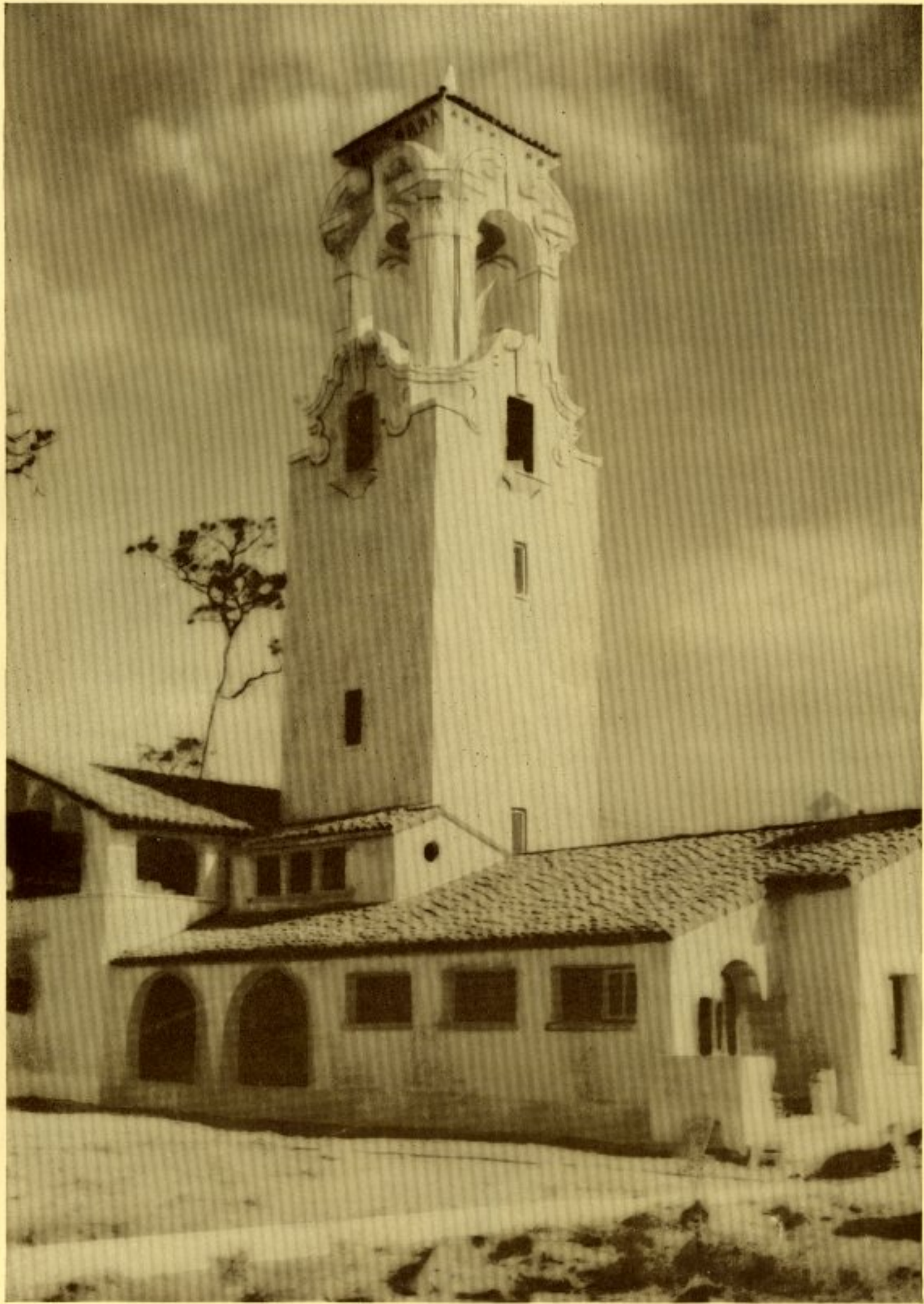
Tower of the Congregational Church of Coral Gables
