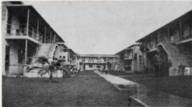
FIFTIETH STREET HEIGHTS apartment project at Northwest 27th Avenue and 50th Street (F). Typical of postwar apartment projects, buildings contain eight apartments each and sites are landscaped. Project has both one and two bedroom apartments, renting for $13.00 and $18.00 per week. Units contain gas stove and six foot refrigerator. Walls are furred and floors are poured concrete. Project was financed by the F.H.A. under Title 608.
