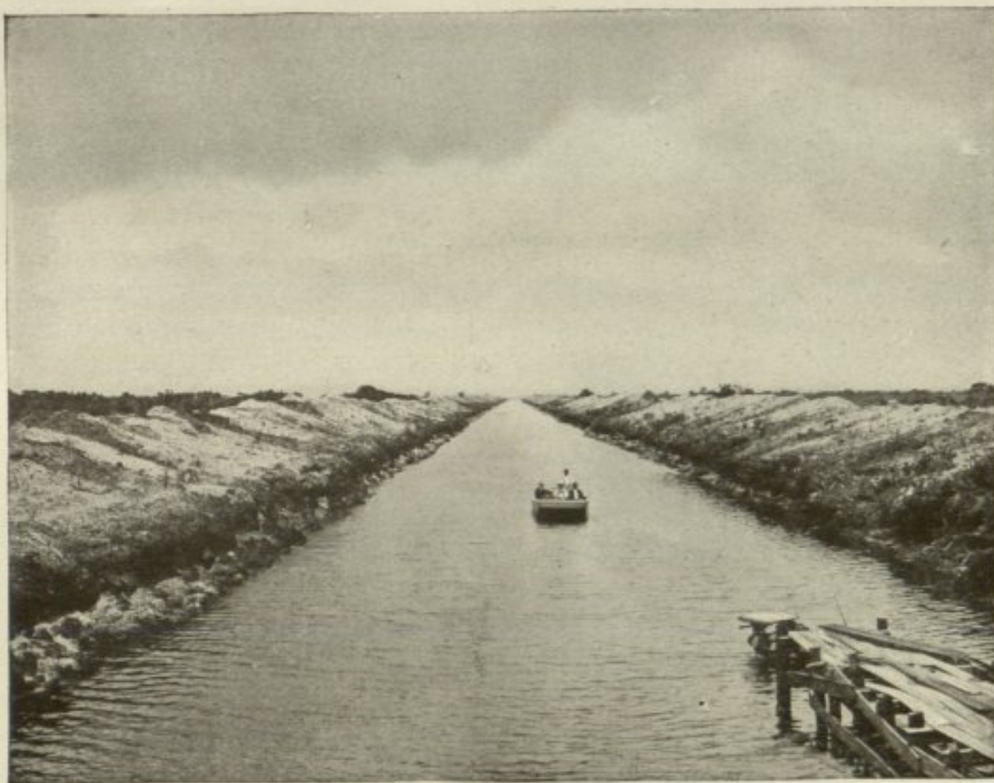
CANAL NEAR EAST RIM.
