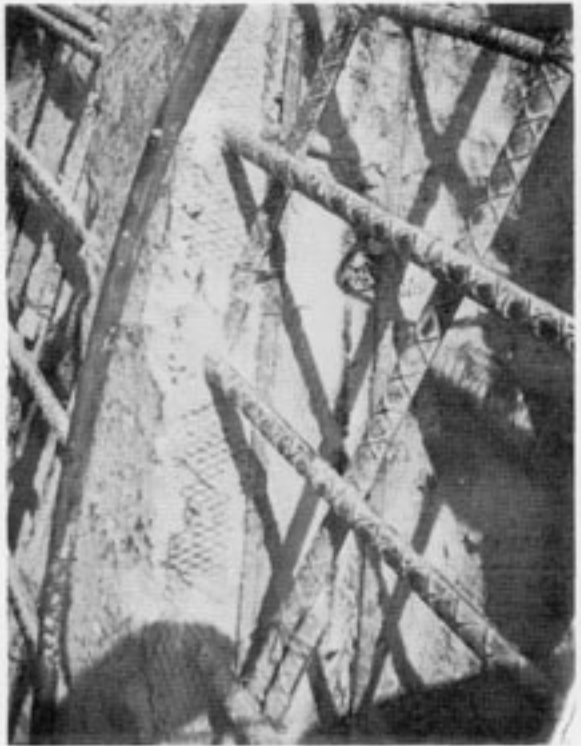
Meridional construction joint 15'-20' south of apex to a depth of 18".
