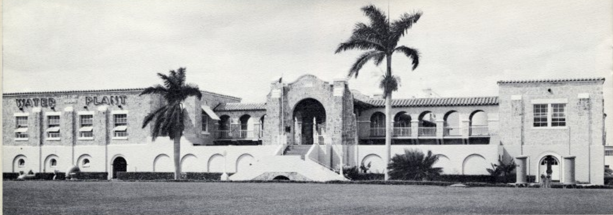
THE HIALEAH PLANT. First built in 1925 and gradually enlarged to a capacity of 80 million gallons a day, it remains a fine example of early Miami architecture utilizing local "oolite" as a facade.
