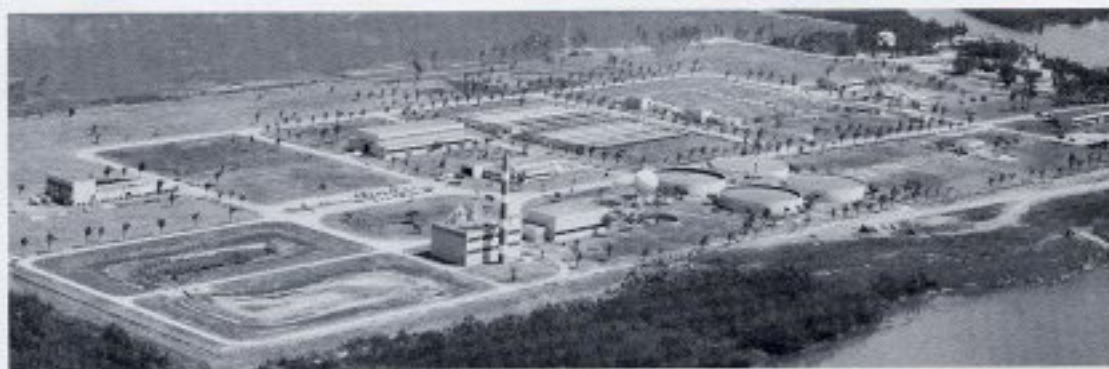
Sewage Treatment Plant
