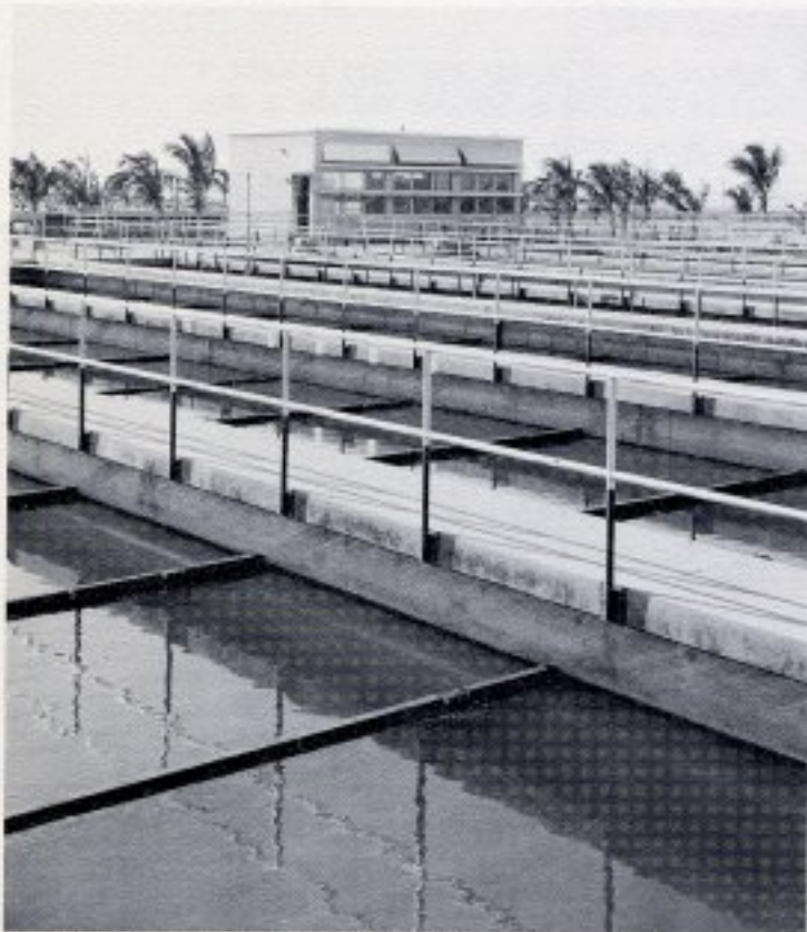
THE TREATMENT CONTINUES. Settleable solids separate from the liquid and pass to the bottom of these settling tanks for removal as sludge.
