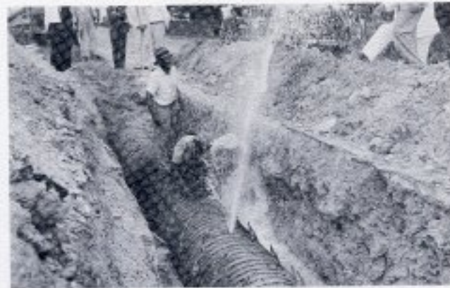
BOOMTIME WOODEN WATER MAINS, 1925 - 1941. California redwood transmission mains were installed from the Hialeah Plant to downtown Miami. The mains were 30 and 36-inches in diameter, made of wood staves fastened together with steel bands. They were short-lived and leaks were many and frequent. They are no longer in service.
