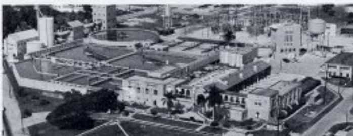
Hialeah Water Treatment Plant
