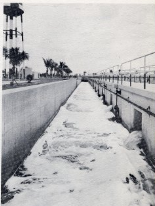
OUT TO SEA. After a final dose of chlorine, all remaining bacteria are killed and the plant effluent is ready for its journey to the sea.
