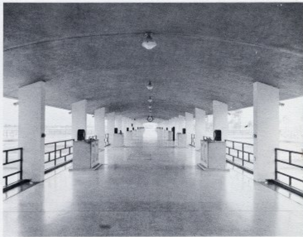
FILTER CONTROLS. The architecturally attractive walkway contains the filter control tables.
