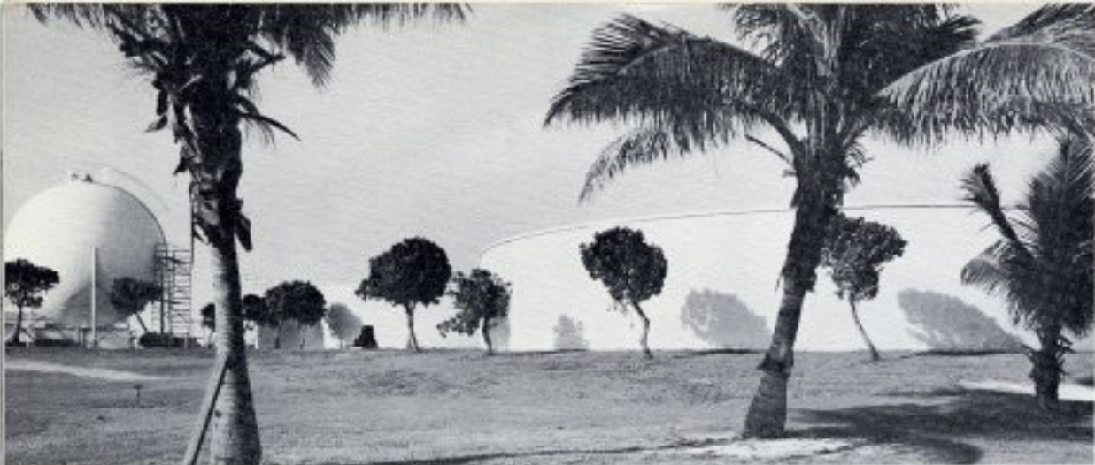
WHERE DO THE SOLIDS GO? Digesters change the solid materials to liquids and gases in 60 to 90 days.
