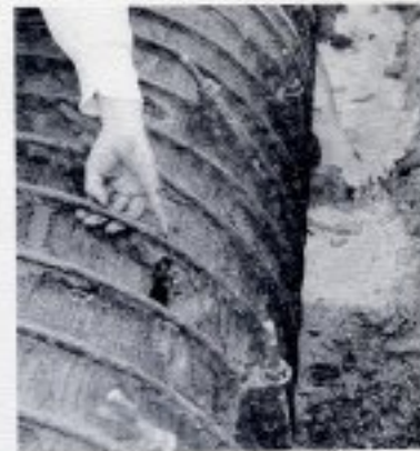
BOOMTIME WOODEN WATER MAINS, 1925 - 1941. California redwood transmission mains were installed from the Hialeah Plant to downtown Miami. The mains were 30 and 36-inches in diameter, made of wood staves fastened together with steel bands. They were short-lived and leaks were many and frequent. They are no longer in service.
