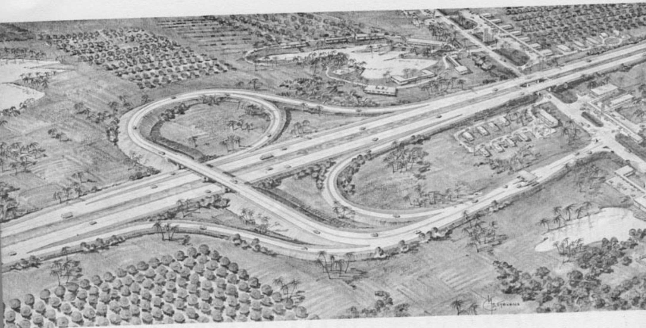
Figure 8. Typical Intermediate Traffic Interchange
