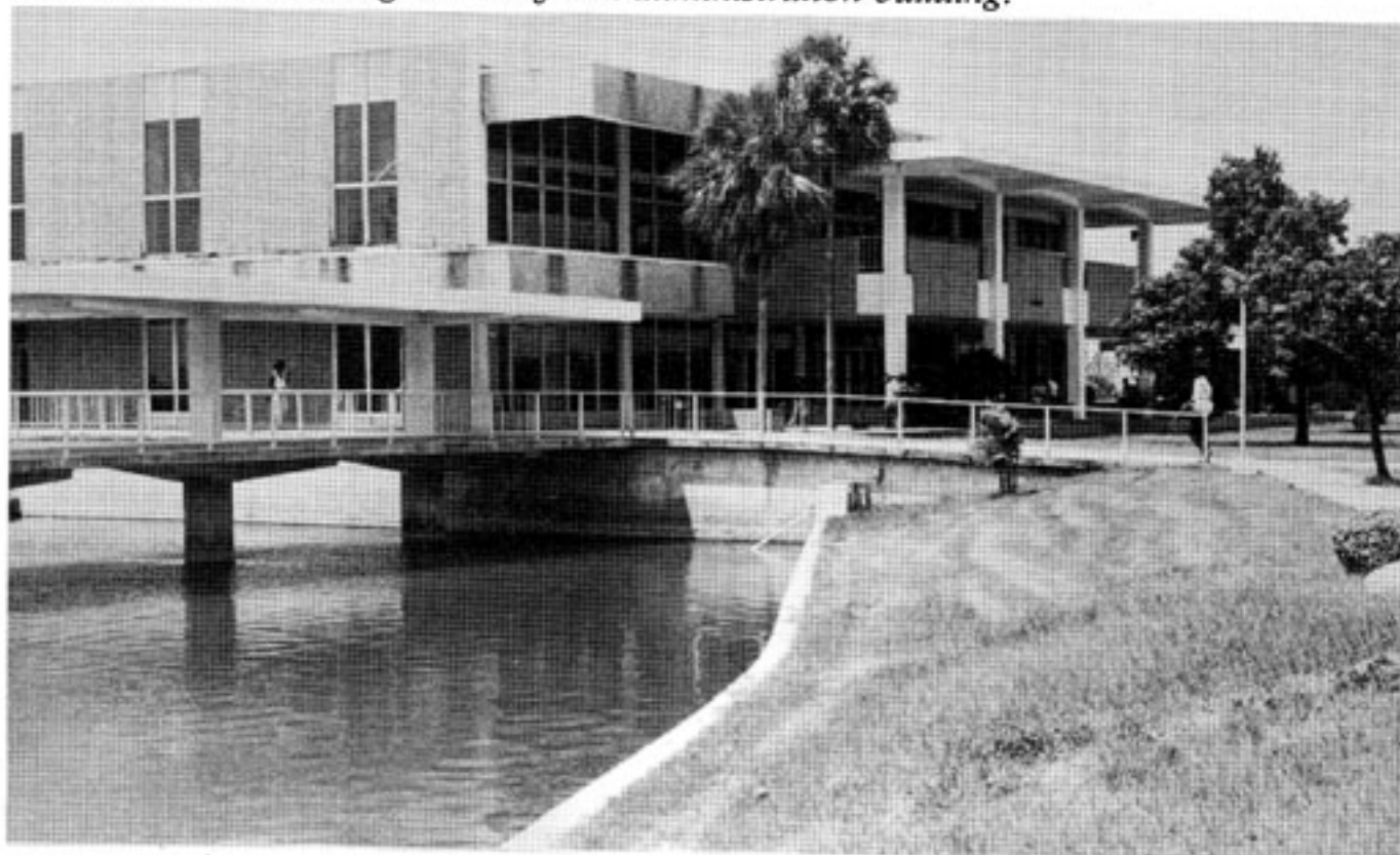
Florida Memorial College's library and administration building.
