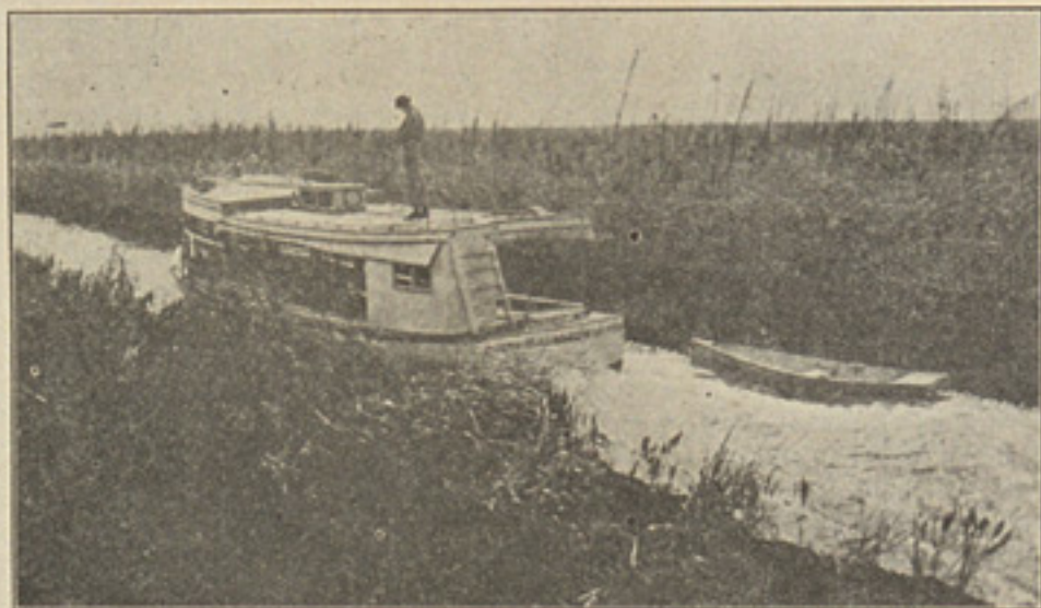
One of the Lateral Drainage Canals
